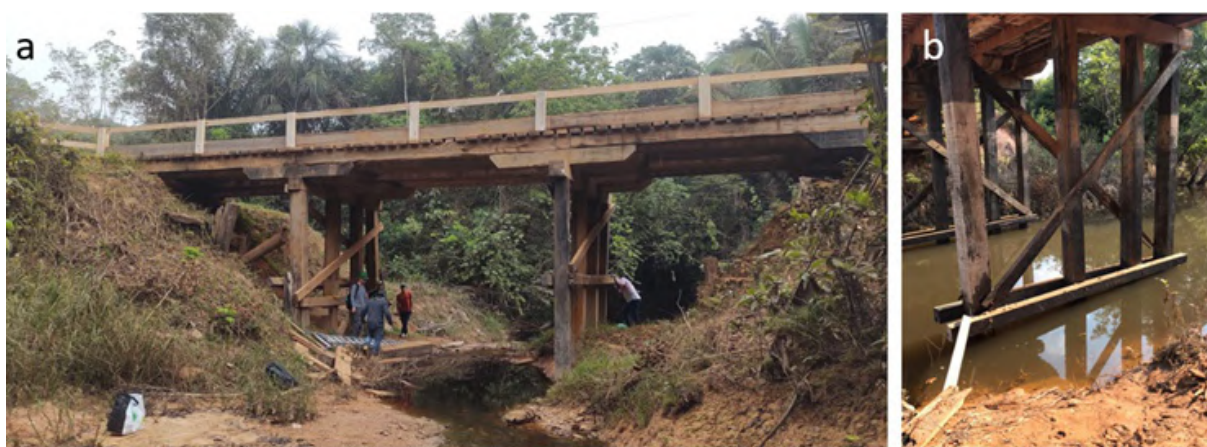
Figure 1. a) Side view of the bridge over the Igarapé Bandeirão; b) Detail of the pillars. Source: Paula et al. (2021)
